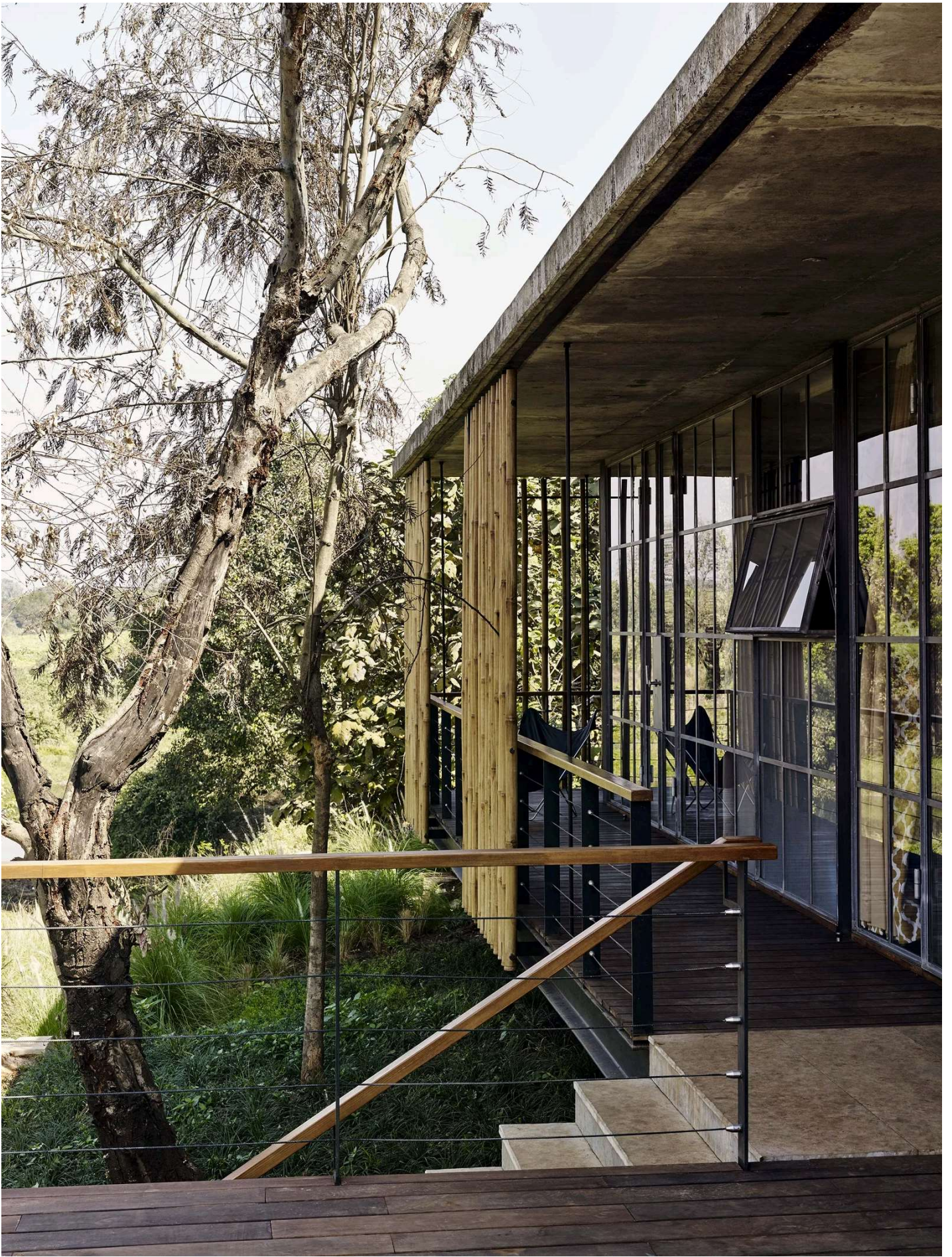
Galvanized steel mullioned windows break down the scale of the front façade of the house.
