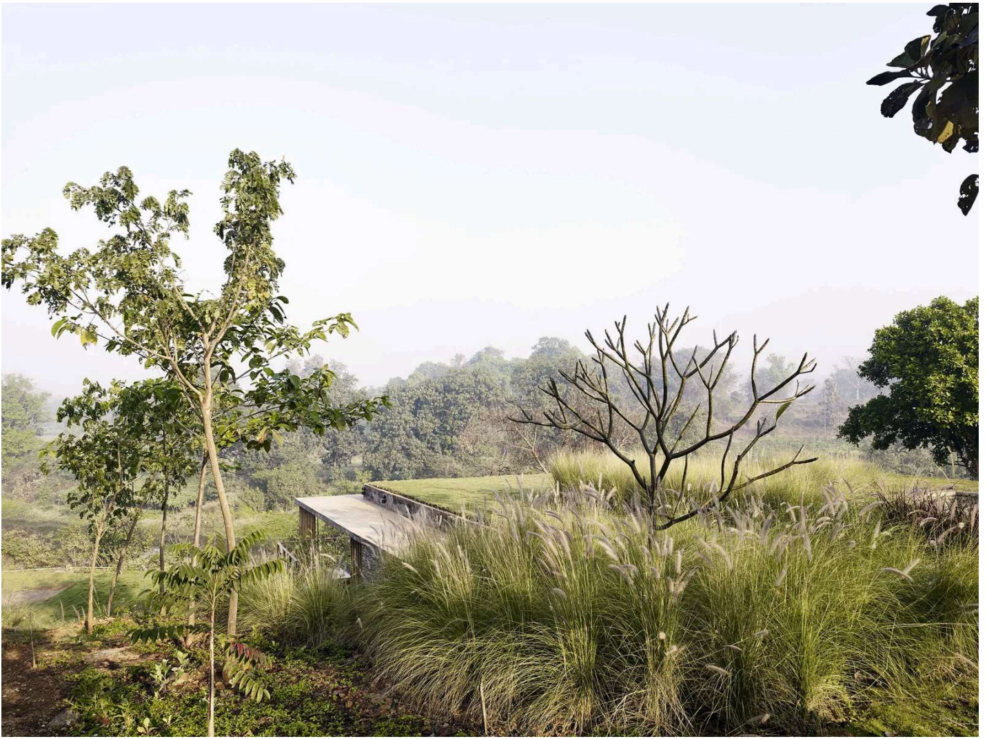
From the top, the roof seems to be an extension of the natural landscape, enhancing the under-statedness of the house. Since the most of the site is steeply sloping with a 1:4 gradient, the vegetated roof gives the subterranean house an additional usable area.
