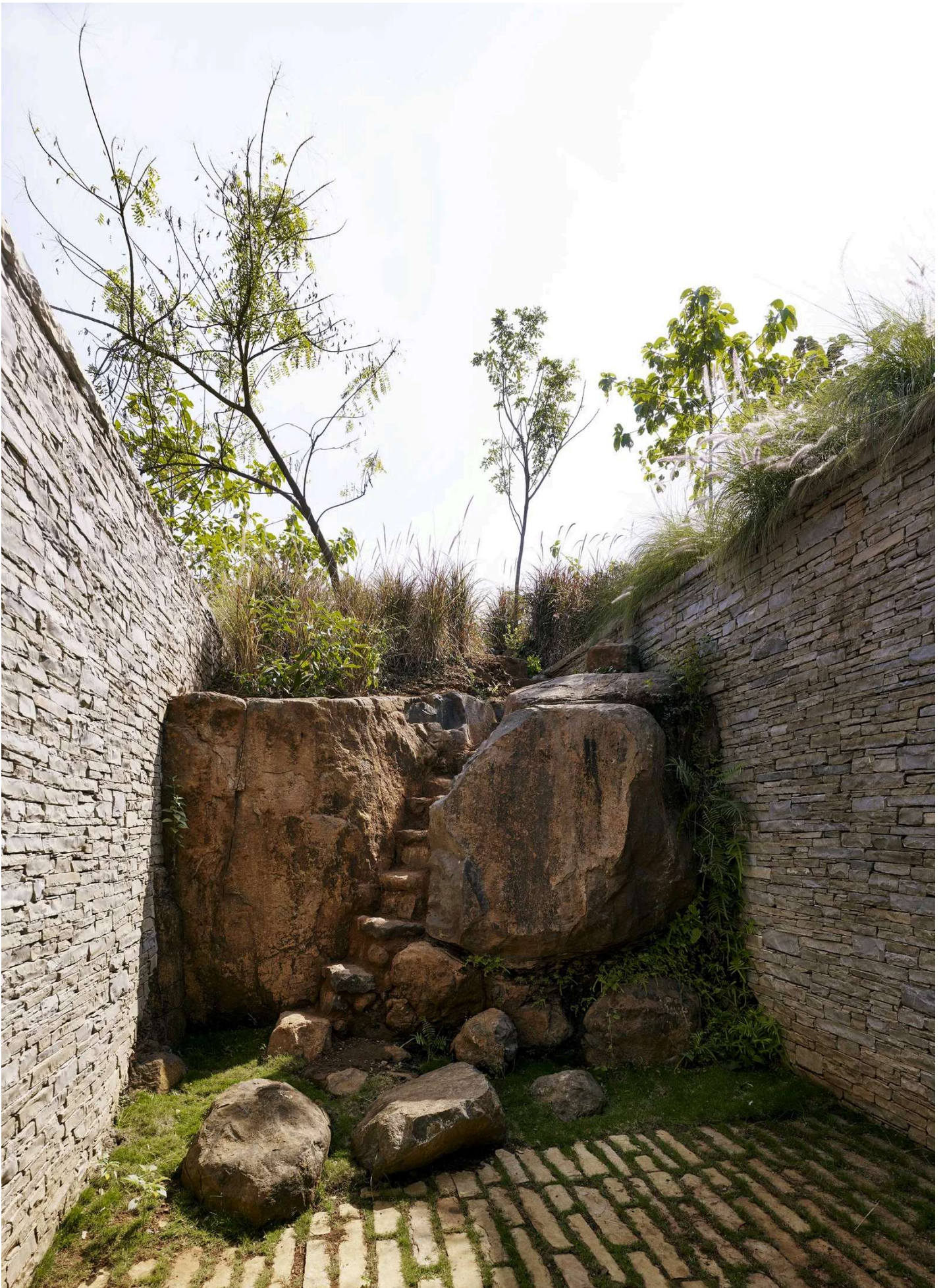
Stone boulders which were discovered during the excavation process and retain the earth.
